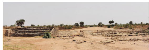
Figure 21. View from downstream of the dam
