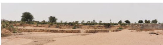
Figure 20. View from upstream of the dam
